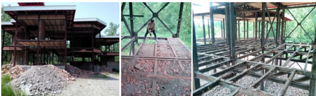
Figure 2. Demolition of the brick arch panel in a steel building to strengthen in Iran
