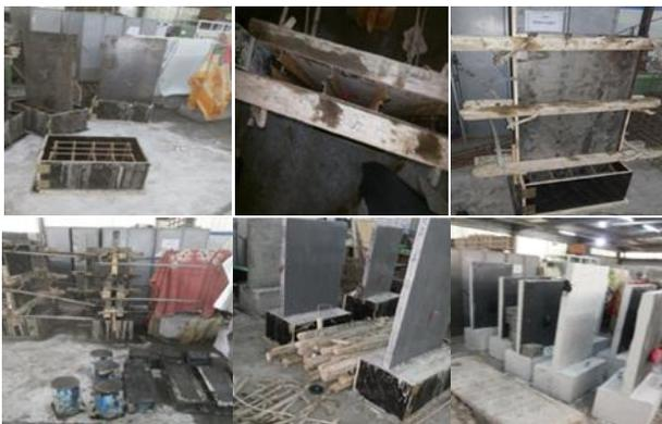
**Figure 6.** The casting of the walls
