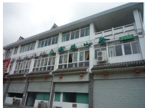
Figure 9 Basically intact BFSWMS
