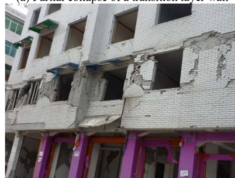
(b) Serious damage to the wall between windows in the transition layer
