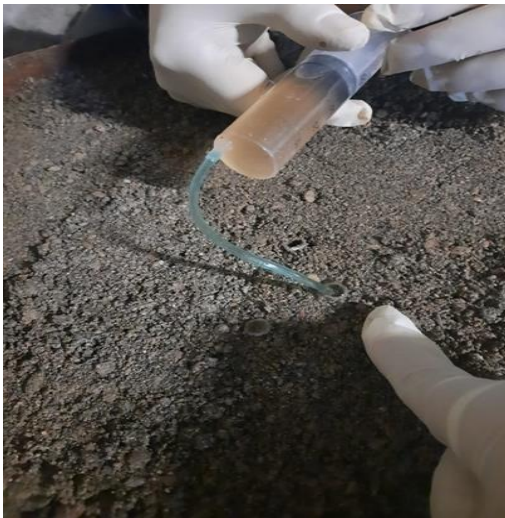
Figure 9. Bio-grout injection in micropile
