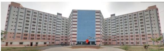
Figure 4. Front view of the 1.8K hostel
