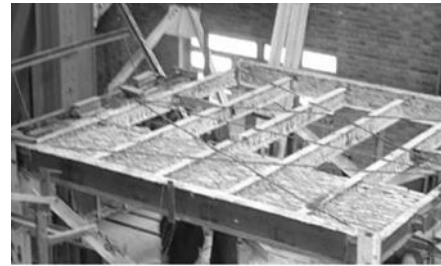
Figure 3. Sample with two X-bracings on the floor slab during construction [4]
