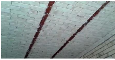
Figure 1. Brick slab after construction
