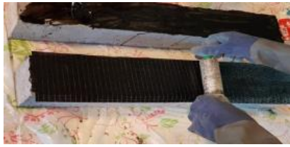
Figure 3. Step of removing trapped air under the CFRP using the roller method
