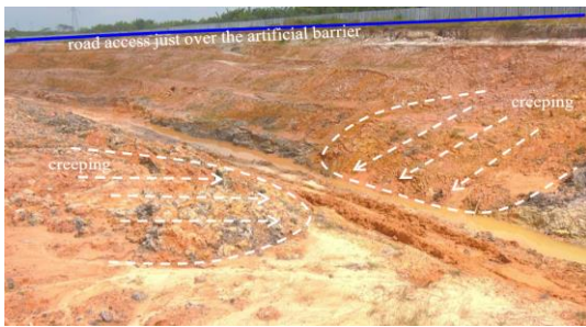
Figure 1. Diversion channel near access road in low water flow condition
