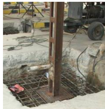
Figure 9. Photo of Foundation Retrofitting
