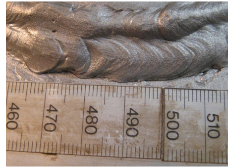
Figure 6. Crack on repaired welded tubular x-joint
