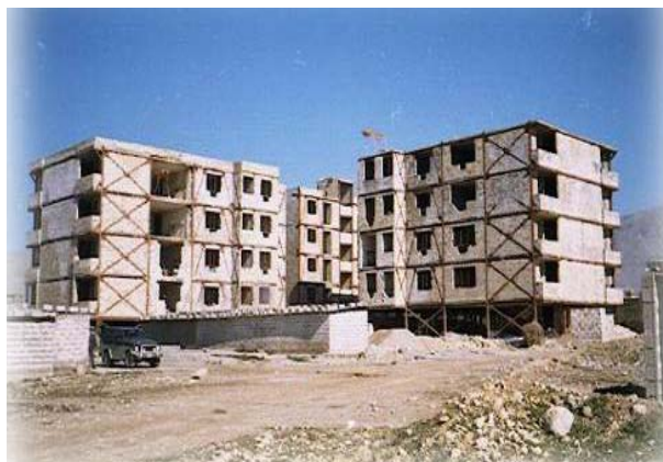
Figure 3. Typical building subjected to evaluation form.
