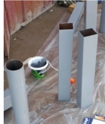
Figure 1. Steel tubes for the CFST columns
