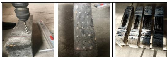
Figure 4. A rough surface for perfect bonding
