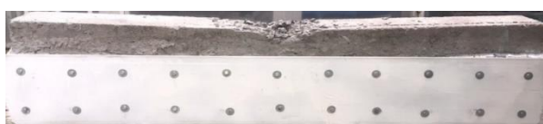
Figure 14. CJ-F2 beam failure mode
