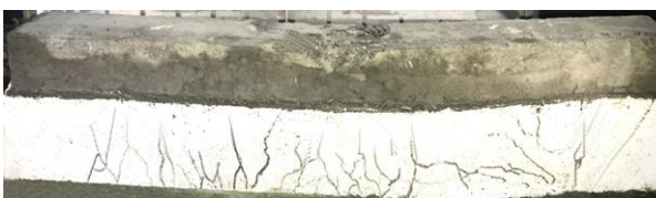
Figure 9. J-F0 beam failure mode
