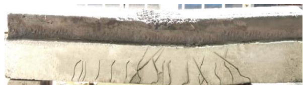
Figure 10. J-F1 beam failure mode
