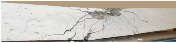
Figure 8. NR beam failure mode
